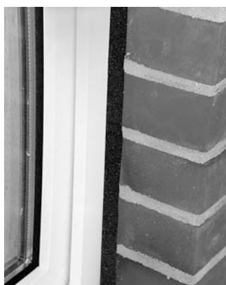
G.U joint sealing tapes are pre-compressed to less than 20 % of the original thickness.
